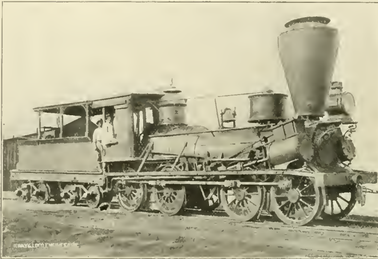
FIG. 79. OLD CUBAN BALDWIN WITH FLEXIBLE DRIVING WHEELS.
